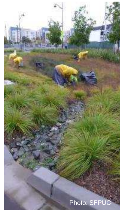
Figure 1. Maintenance of bioretention facility.
