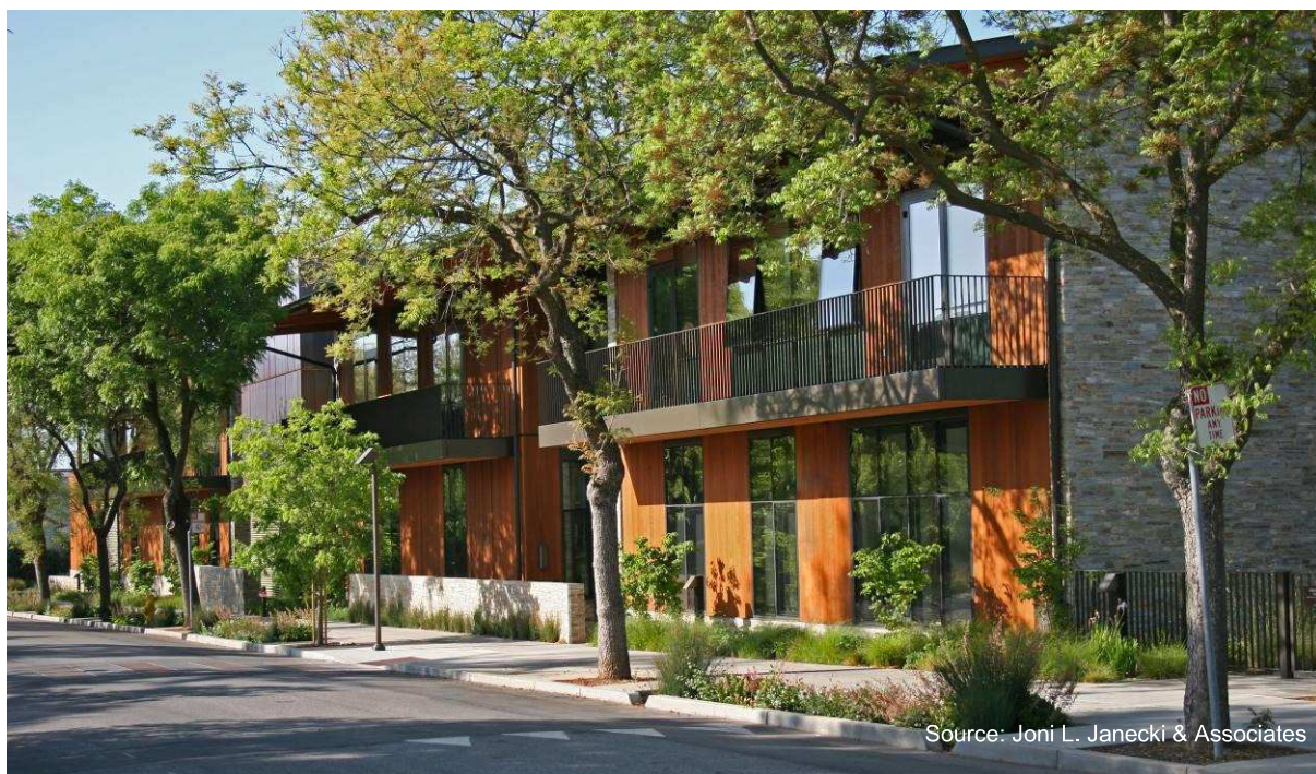
Figure 2. In this Los Altos project, curb cuts direct street runoff to vegetation. Downspouts are directed to cisterns and swales.
