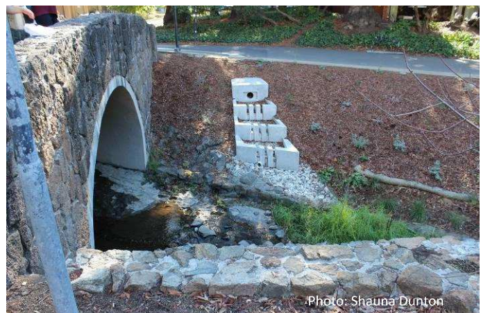
Figure 3. Energy dissipation, erosion control, and stream buffers at Strawberry Creek in Berkeley, CA.
