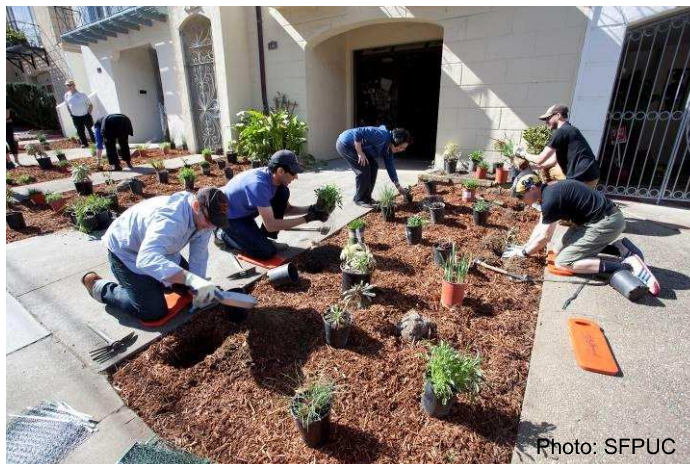
Figure 3. Disconnecting downspouts, removing impervious surface, and installing native plants in San Francisco, CA.
