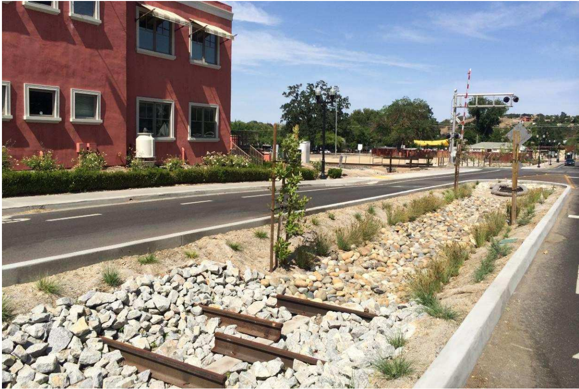
Figure 2. Railroad rails and rip rap to slow stormwater flows in a creek daylighting project in Paso Robles, CA.
