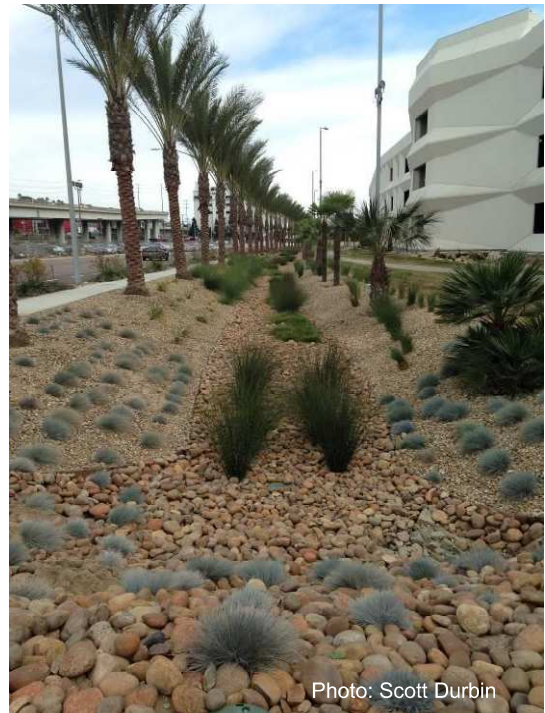
Figure 1. Swale at San Diego Airport with rock mulch, low-water plantings, and irrigation controls.
